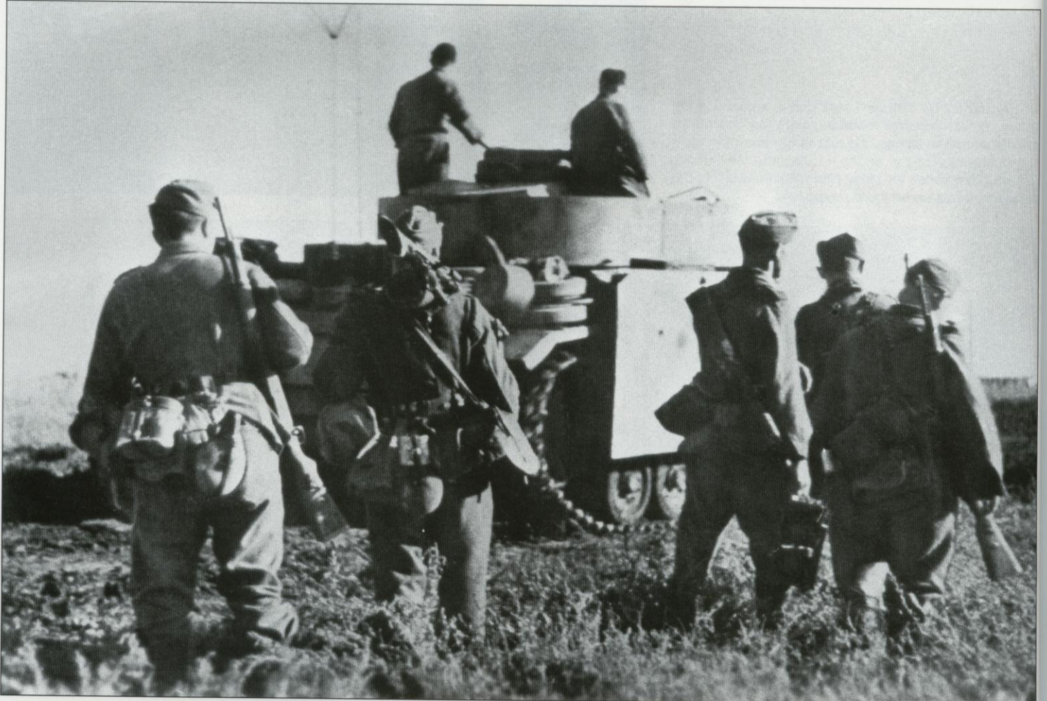
Soldiers support a Pz.Bef.Wg. III Ausf. K. Operation "Zitadelle" was the last battle in which this type of tank was used in large numbers. There were around 50 vehicles of this version produced from December 1942 to February 1943. By late 1943 it had become obsolete.
